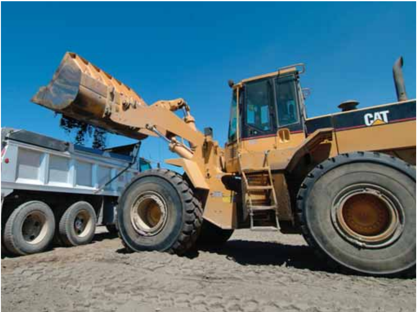
► RUSH SITE PREPARATION PUTS 970F WHEEL LOADER TO WORK
